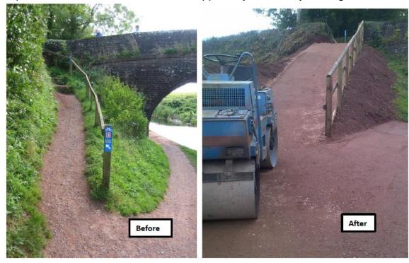
Contractors then used an excavator to re-profile the hedge bank and create the ramp, and then surfaced the ramp with limestone scalpings and compacted them with a vibrating roller. A handrail was also installed. A post and rail fence along the field boundary is due to be installed by a fencing contactor in the next week. The Canal Ranger wishes to thank the adjacent landowner, Mr Venner, for his assistance in providing access for the works.
