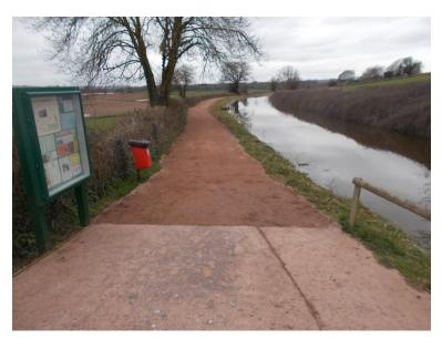
In general the width of the surfacing is a bit greater than is usually undertaken, as repairs had to be made to ruts created by the dumper which ferried hundreds of tonnes of stone along the section. A dozen or so gullies between the towpath and the water were also filled in using large rocks and soil.
