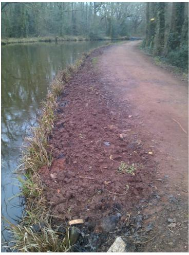
The coir rolls were preestablished with Pendulous Sedge (Carex Pendula) which our botanical advisor (Jeremy Ison) agreed would be suitable as it is common locally and is tolerant of shady conditions. Soil was being used to backfill between the bank and the coir rolls.
